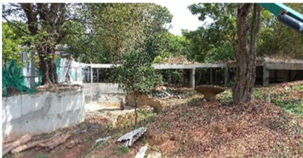
Renovation of the Lion den at Dehiwala Zoo
